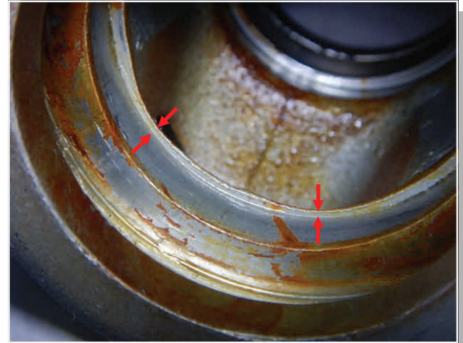
Ph (4) - FH - Seal Housing - Replaced - Seal groove wall damaged, will not hold wear strip.
